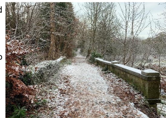
Murieston Bridge – listed
